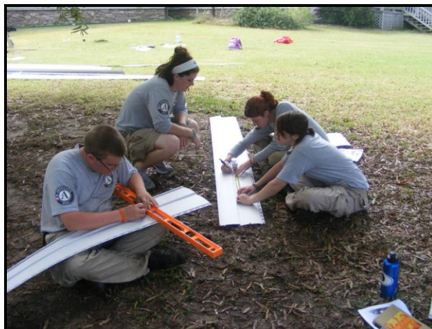
Cut corner vinyl siding so that it fits atop the tower.
