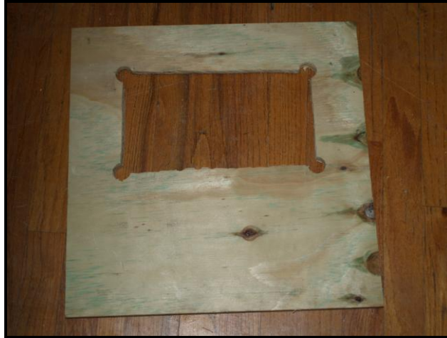
A sun collar platform with a hole for the Chimney Swift to enter. A wood-boring bit was used in each corner to allow a hand saw to cut out a (relatively) straight line.
