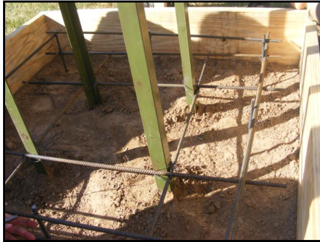
A foundation pattern with rebar installed.
