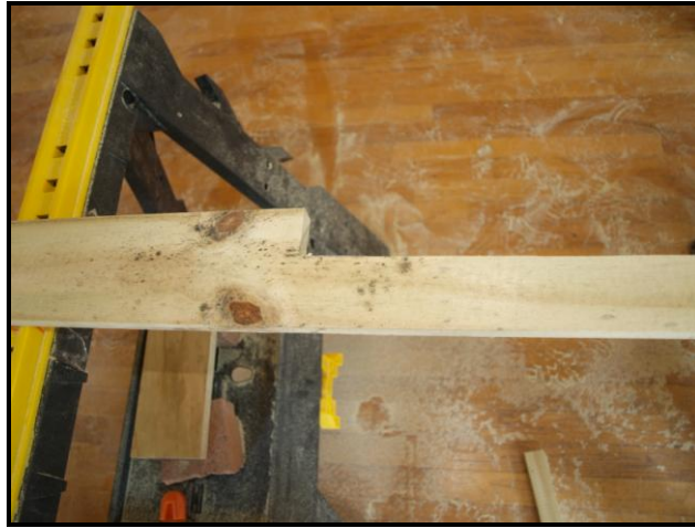
A six-foot 1" x 4" brace with a 1 1/2" x 4" section notched out of it.
