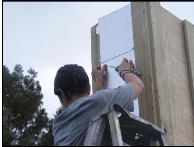
Use direct pressure to attach the siding.
